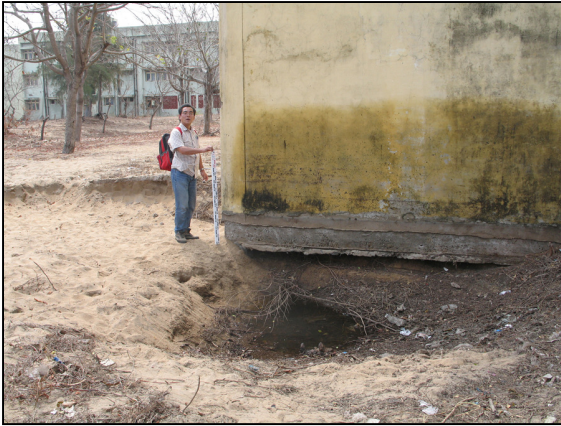
Scour depth 1.2 m
