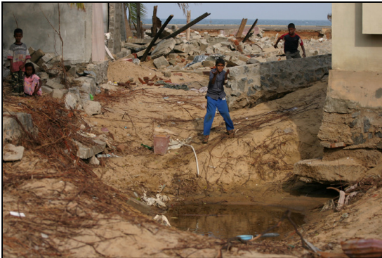
Scour depth 2.0 m
